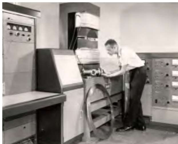
Mass Spectrometer Used to Improve Isotopic Analysis of Process Gas
